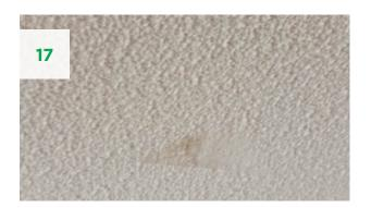
This area was damaged by a door. The impression goes deep into the surface and it flattened the area around it.
