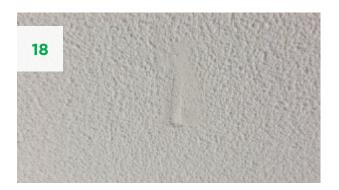
This is another blemish in the ceiling caused by contact with a door. The surface was flattened out and lost all its texture in the damaged area.
