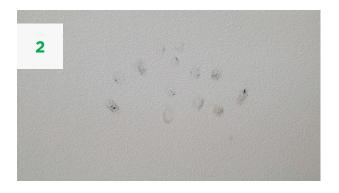
Dirty finger prints on the finished ceiling is one common issue requiring maintenance.
